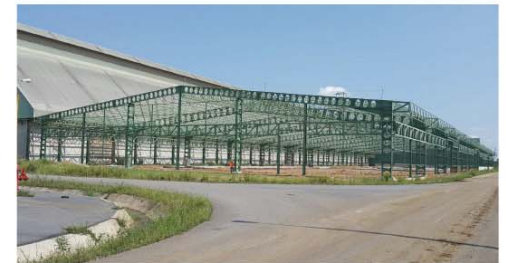
Material Warehouse , Chachoengsao
